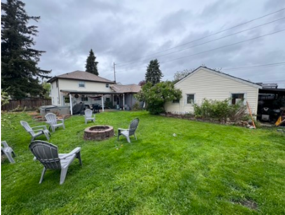
The photo above faces to the north and shows the rear of the existing detached garage and residence.
